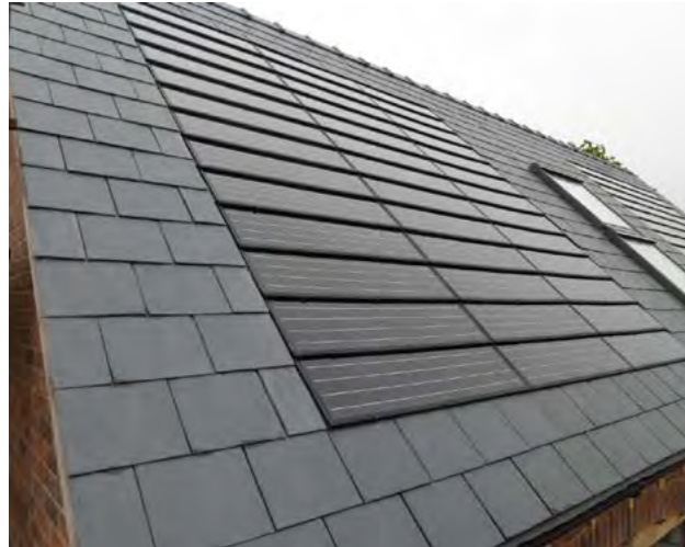
Figure 34: Integrated solar panels on slate roof.
