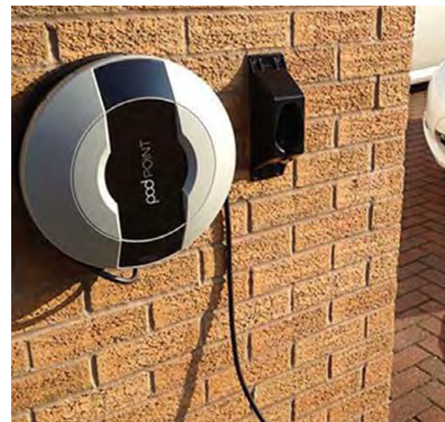
Figure 38: Home electric vehicle charging point.
